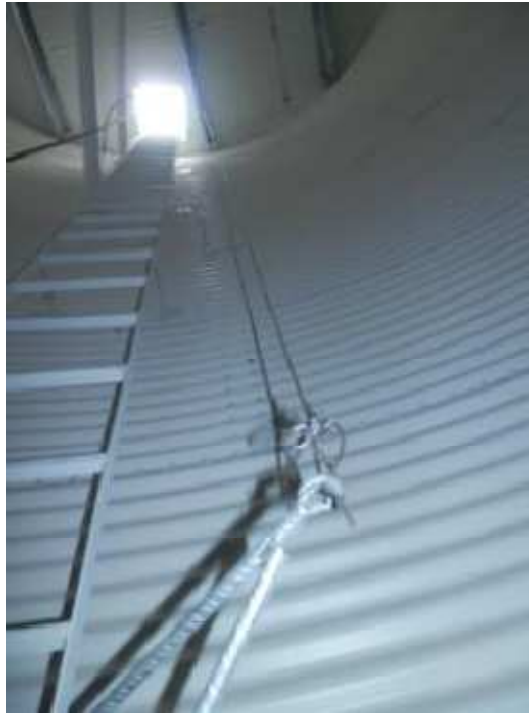
Monitoring of tank temperatures
