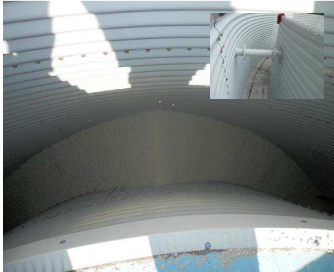
Granular PU between tanks (lateral and upside)
